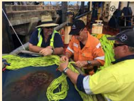
Ardent Senior Salvage Officer, David Skola (centre), splicing a connection link into a 52mm emergency tow line during a training session.
